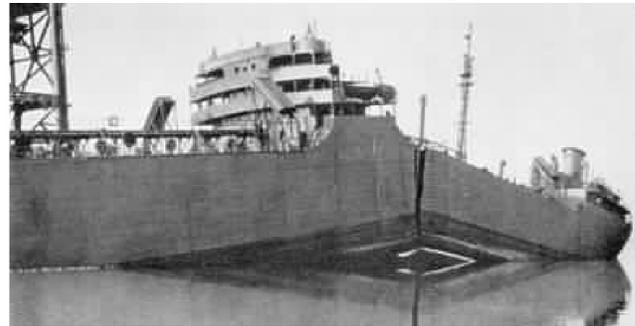
Tanker S.S. Schenectady fractured a day after its launch in January 1941<sup>3</sup>.
